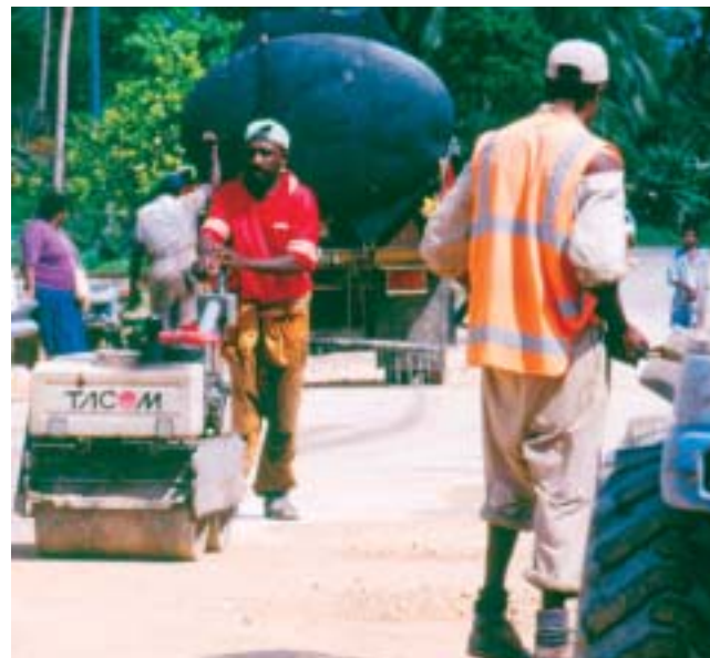
ADB-funded road construction.
